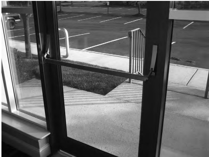
FIGURE 5.54 A push bar (also known as crash bar or panic bar) installed to comply with fire codes.
