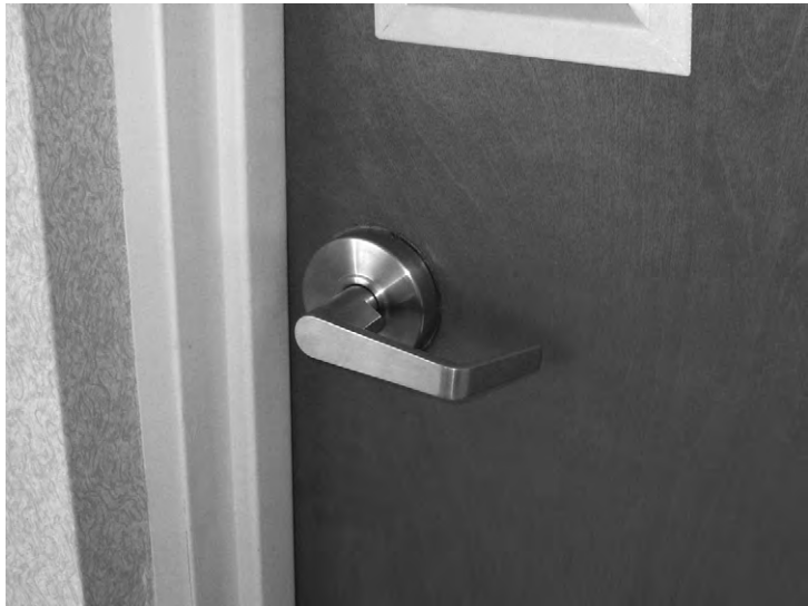
FIGURE 5.53 An ADA-compliant door handle.
